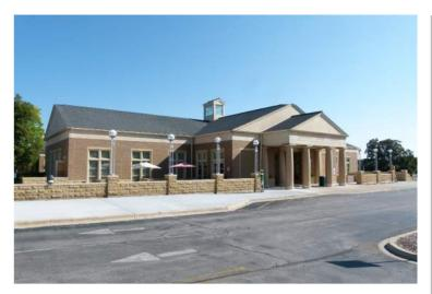
The Batavia Public Library is a 2-story, 54,000-square foot library facility completed in 2001. Sitework components around the building included cast-in-place concrete sidewalks and stairs, cast stone-clad grade separation walls, steel guardrails and handrails, and decorative column covers.
